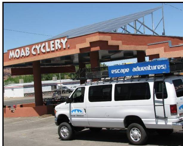
High-visibility solar panels on Escape Adventure’s bike shop, Moab. (Photo courtesy of Jared Fisher)
