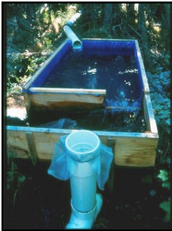
AWA's "low drop, high flow" hydroelectric system. (Photo courtesy of Kirk Hoessle)
